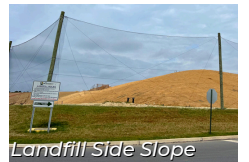
Landfill Side Slope
