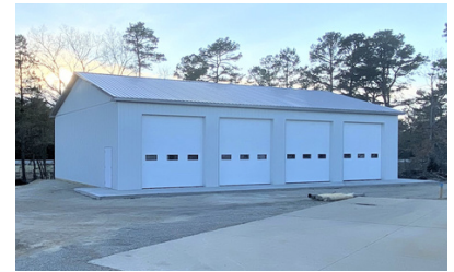
RCSJ Maintenance Storage Building
