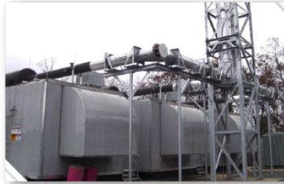
3 Landfill Gas Engines
